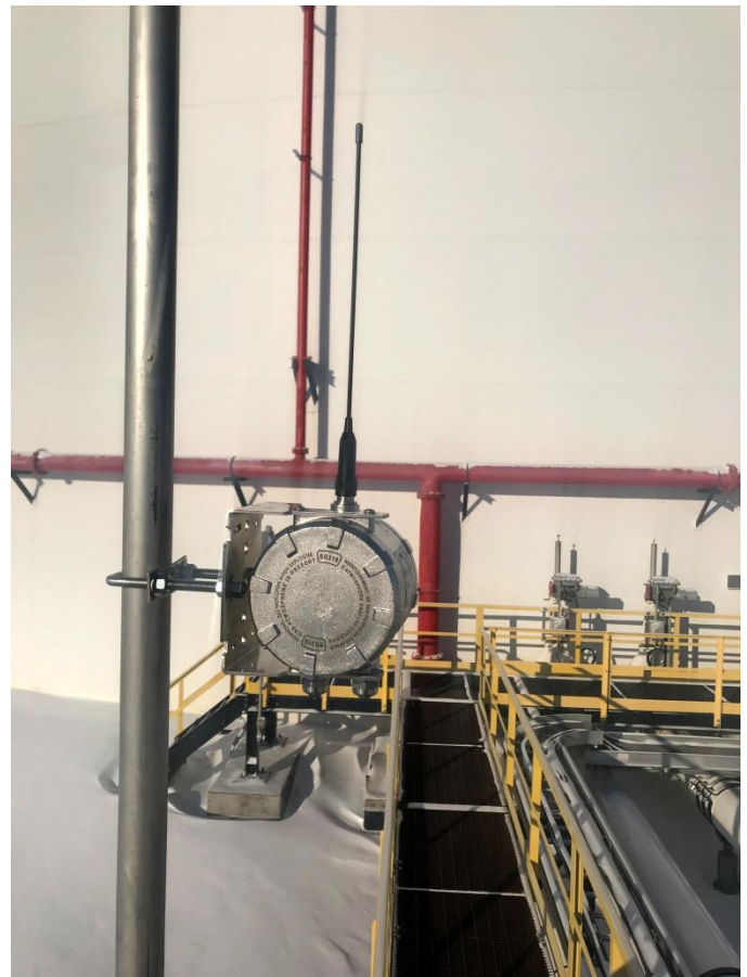
Syscor's PCU-X00 Repeater mounted to an existing pole with the Universal Mounting Bracket and U-bolt.
